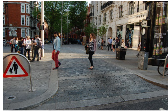
Crossing with similar material to the pavement to act as a traffic calming measure
