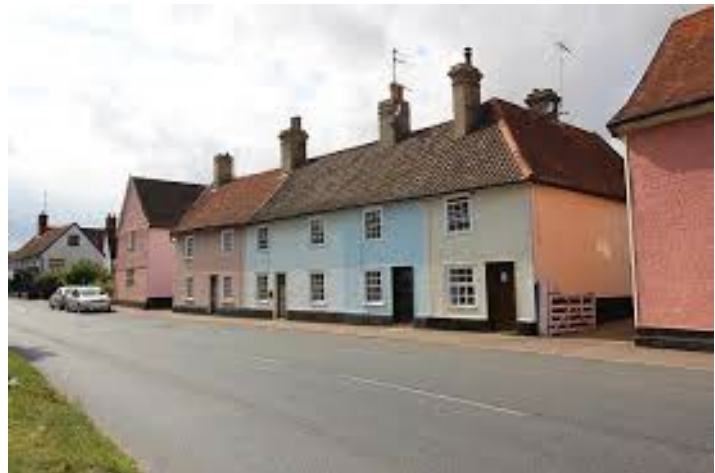
Figure 4.2 Traditional Suffolk style using steeper pitch roof, pantile, brick and coloured render
