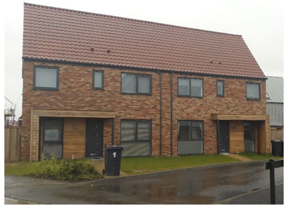
Figure 4.6 Example of a steep-pitched roof on a modern design of property that is not out of keeping with tradition
