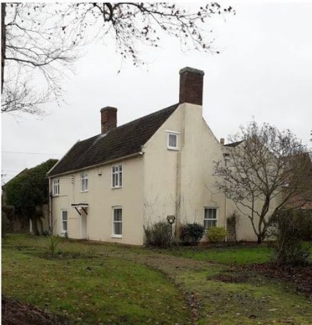
Figure 4.1 Many old buildings exist in the community - Bell Farm
